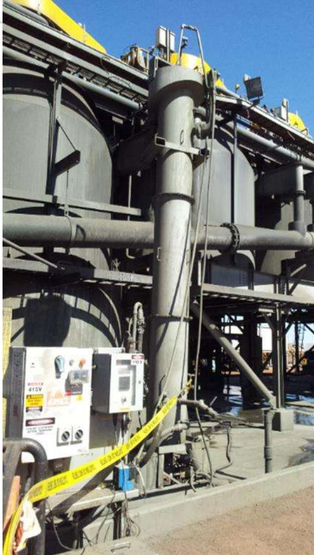
500 mm pilot unit at site
